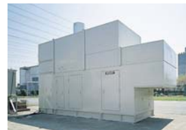
Cogeneration system (combined heat and power system)
