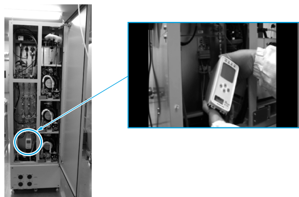
Fig. 4 View of Ozone Sensor Replacement
