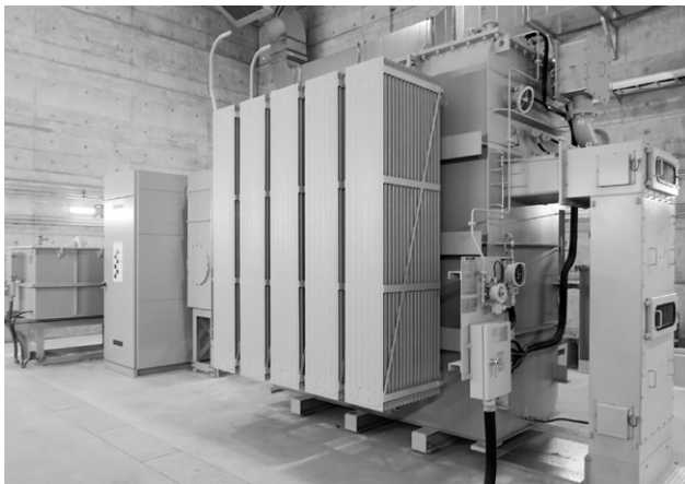
Fig. 7 Main Transformer
