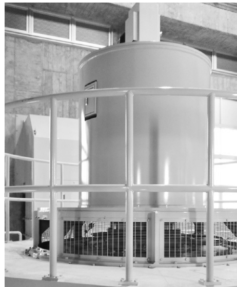
Fig. 3 Runner Vane Servomotor
