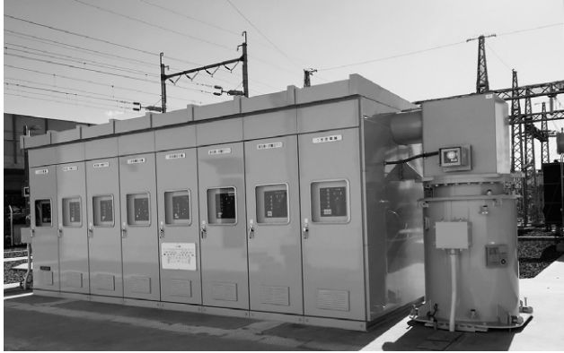
Fig. 9 72 kV Outdoor Type C-GIS
