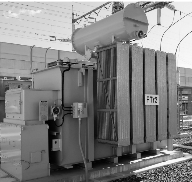
Fig. 5 Scalene Scott Connected Transformer
