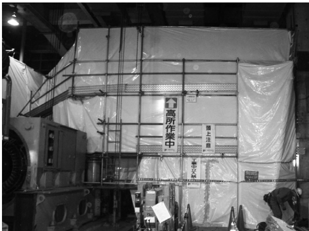
Fig. 7 Removal of Asbestos from Turbine Engine
