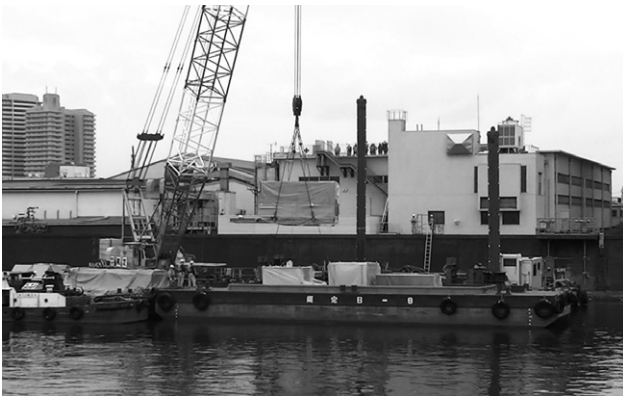
Fig. 16 Generator System Transportation by Barge
