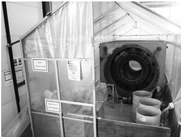
Fig. 8 Removal of Asbestos from Generator Main Body
