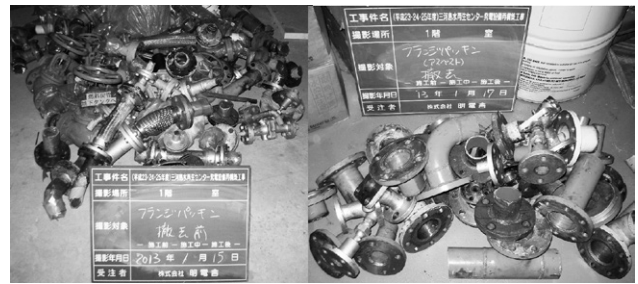
Fig. 9 Removal of Asbestos from Flange Gaskets of Fuel Pipes
