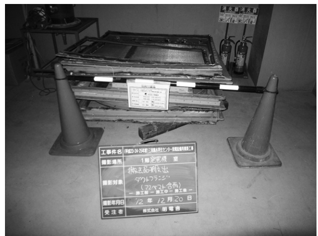
Fig. 10 Disposal of Flange Gaskets from Air Conditioner Ducts
