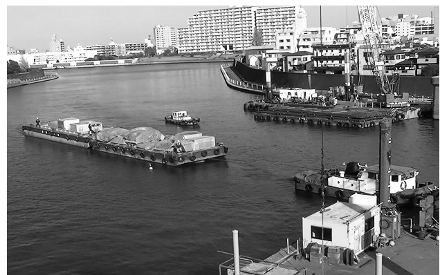
(b) A view of transportation near the pumping station
