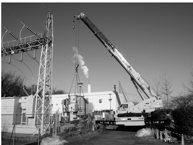
Fig. 4 Crane Work during Carry-in and Carry-out Period
