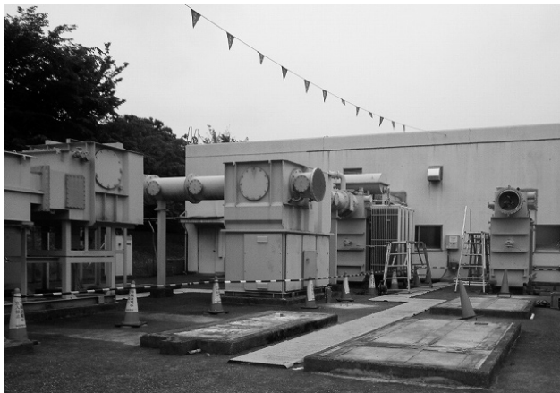
Fig. 3 Work Situation near Renovation Construction Work
