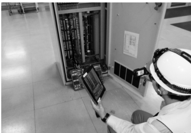
(b) A view of checking the work done
