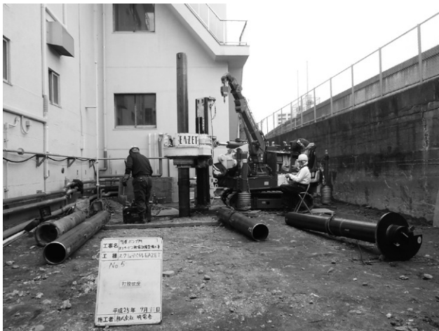
Fig. 14 Piling Work for the Generator Foundation
