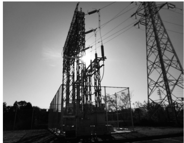
Fig. 4 View of Gate-Shaped Lead-Line Steel Tower
