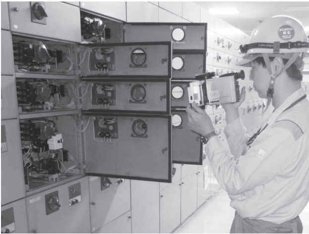
Fig. 2 Situation of Thermographic Diagnosis
