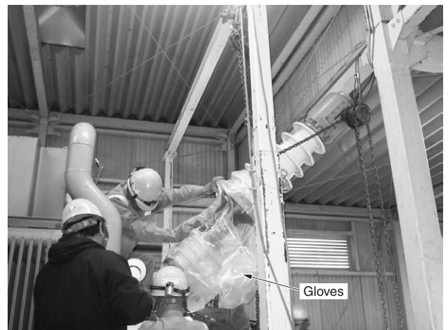
Fig. 3 Parts Removal Work (for a bushing)
