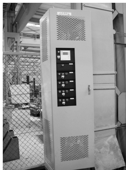
Fig. 2 Installation Example of Automatic Low-Voltage Power Factor Controller
