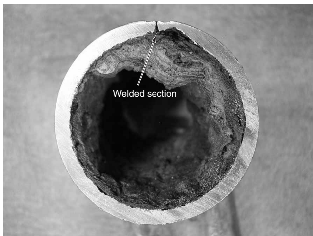
Fig. 4 Cross-Section of a Cooling Pipe Suffering from Corrosion
