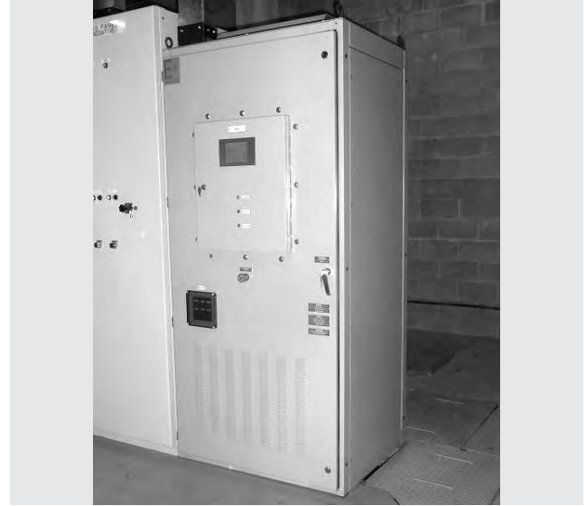
Fig. 7 Outline of AARU Controller Outline of AARU controller equipped with thyristor switches.
