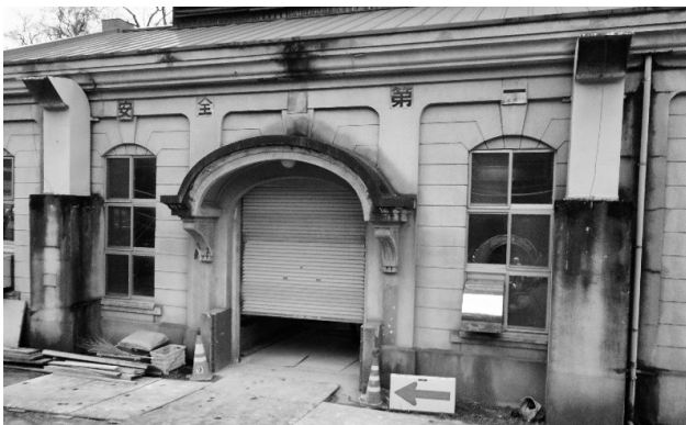
Fig. 6 Carry-in Entrance of Existing Plant Building
