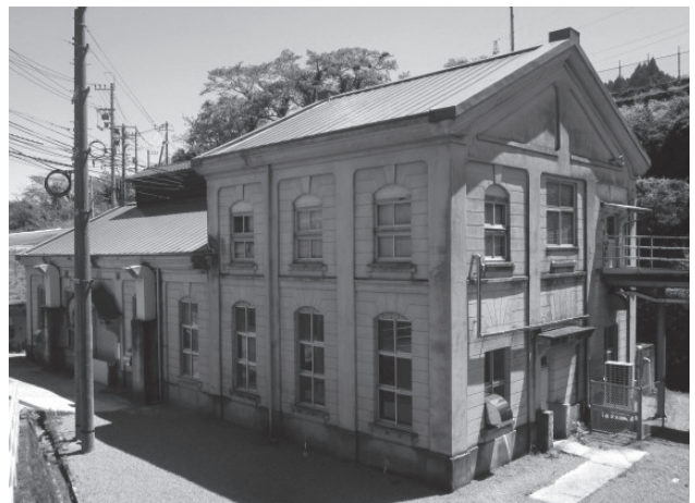
Fig. 1 Panoramic View of Asahi Power Plant Building
