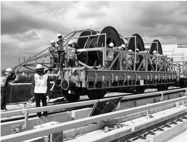
Fig. 3 View of Cable Laying Work
