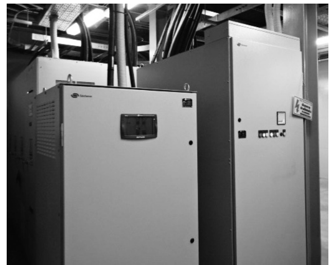
Fig. 12 VLD (Left) and Cathode Panel (Right)
