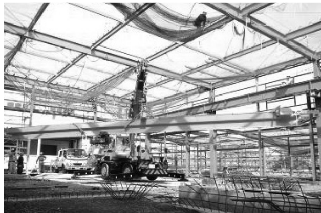
Fig. 3 Installation Work for the Product (Pipes) Conveying Overhead Traveling Crane
