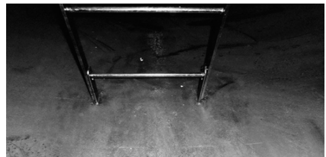
Fig. 5 Tank Inside after Cleaning
