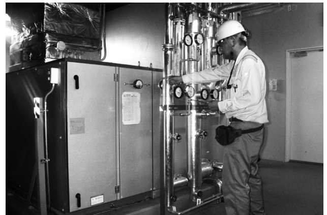
(a) Routine inspection for an air-conditioning facility
