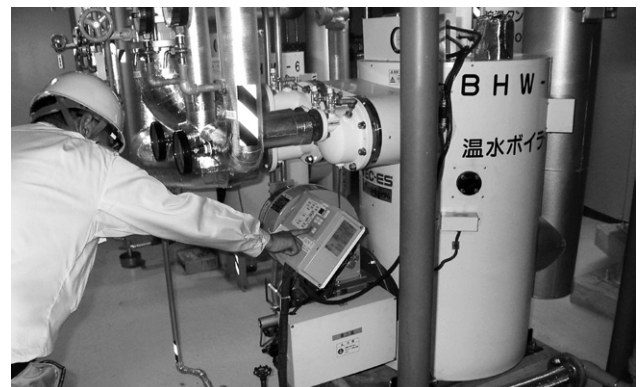
(b) Routine inspection for a heat source facility
