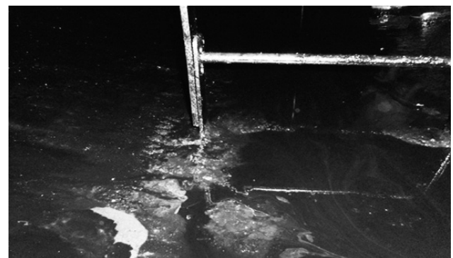
Fig. 4 Tank Inside before Cleaning
